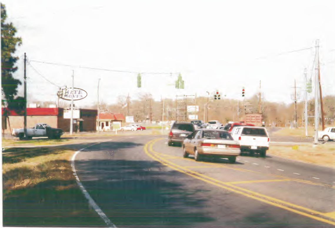
Choctaw/Flannery Intersection, South Approach Note Flannery superelevation, curvature on approach
