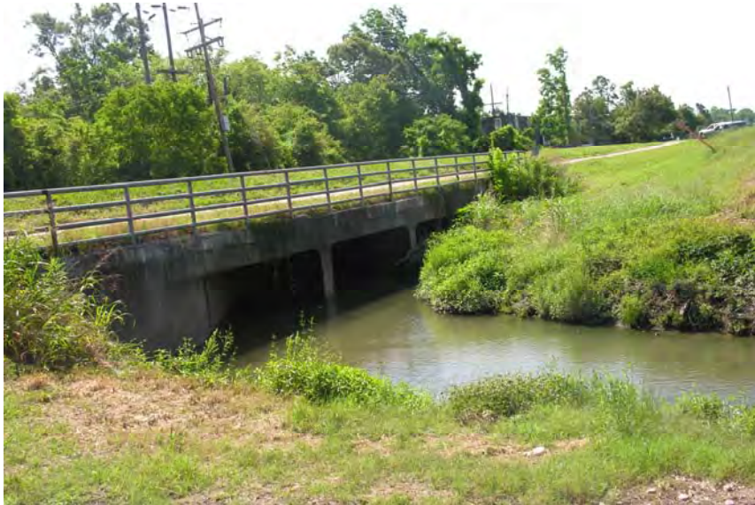
Figure 4: Picture of (3) RCBC’s at Sta. 307+13 taken by Jason Ellis May 9, 2009
