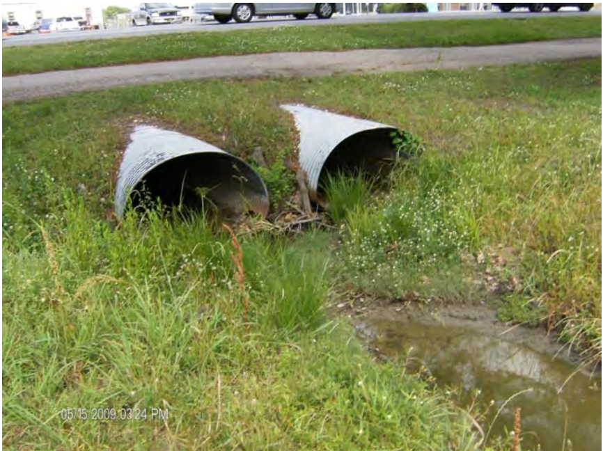
Figure 6: Picture of (2) 36” CMPA’s at Sta. 346+10 taken by Jeff Diamond May 15, 2009
