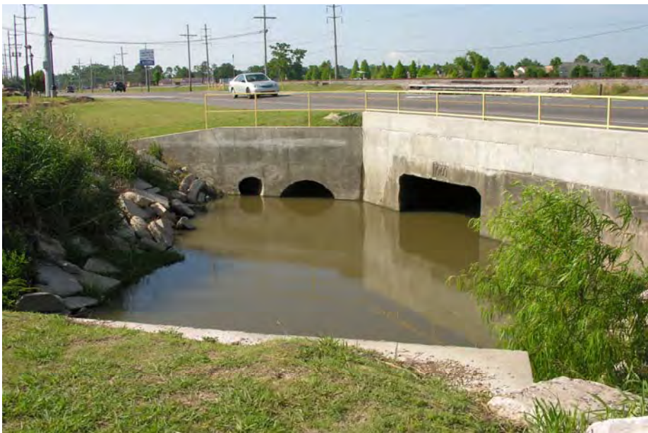
Figure 5: Picture of 8’ X 8’ RCBC and 84” steel culvert at Sta. 337+56 taken by Jason Ellis May 9, 2009
