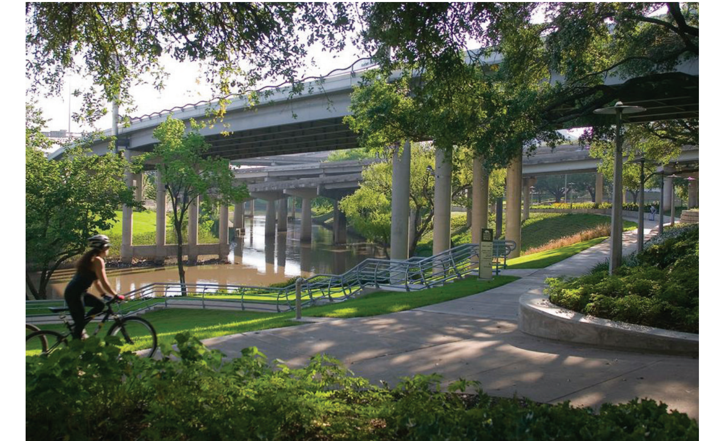
(B) UNDER THE BRIDGE
