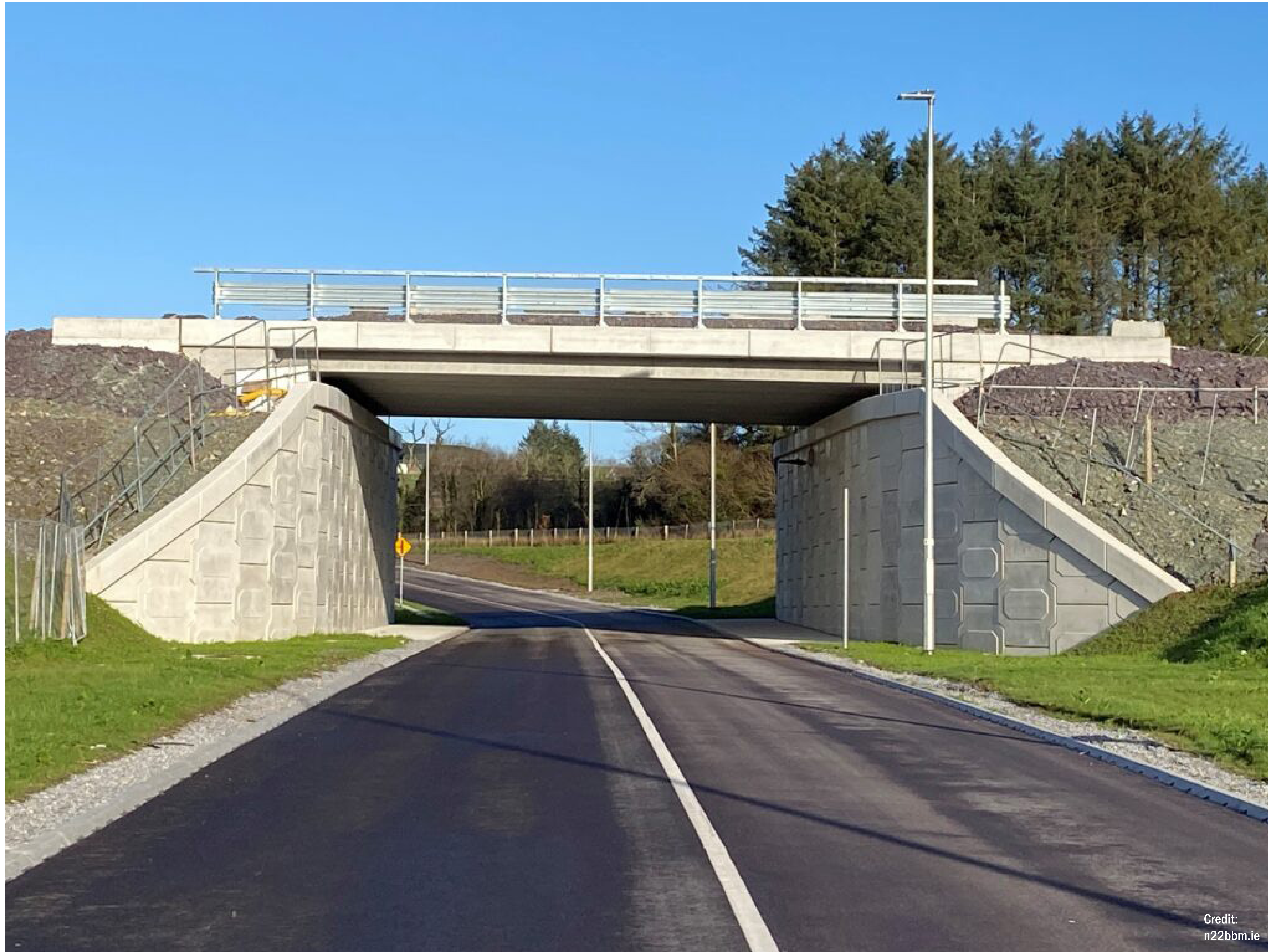
MSE (Mechanically Stabilized Earth) Wall - Example Photo
